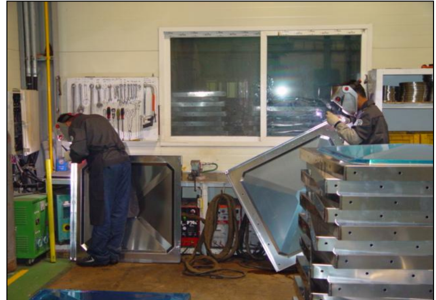
Welding of Panel Conner – 2
